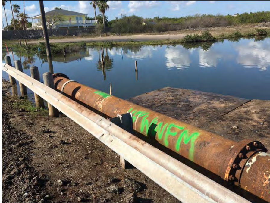
29. The pipe from the previous photo can be seen. It appears to be a wastewater force main.
