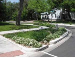
Example of Bioswale Drainage
